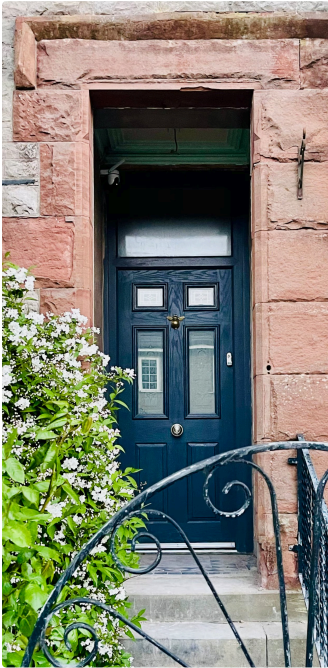
The front door, in red sandstone.
