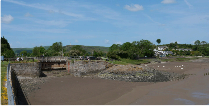
The sea lock and pier at Canal Foot.
